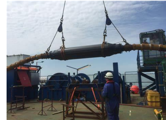
Cable Joint on Vessel
