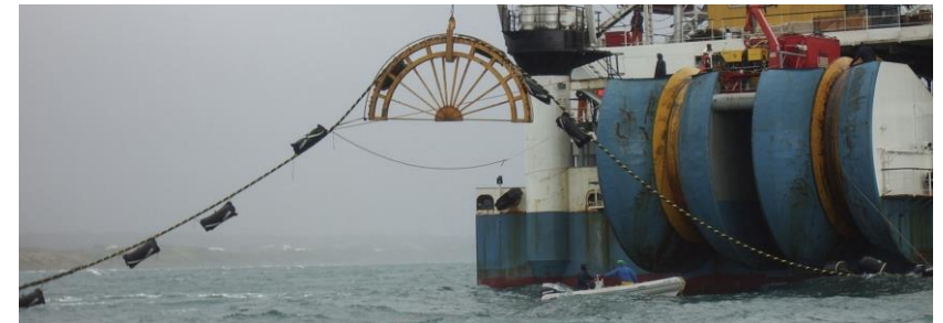
Export Cable Laying Vessel
