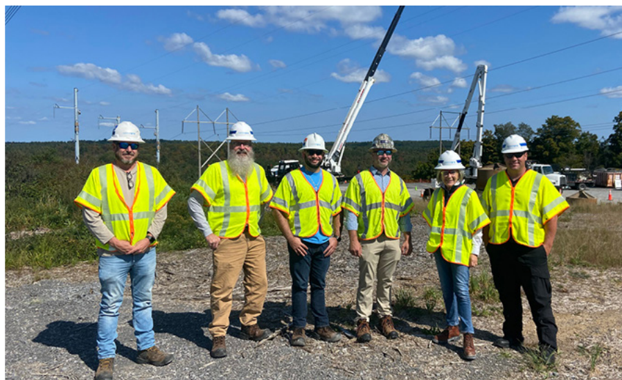
Paula Rosput Reynolds visiting our Smart Path Connect Project near Boonville, New York, which is an under construction 345 kV transmission project.
