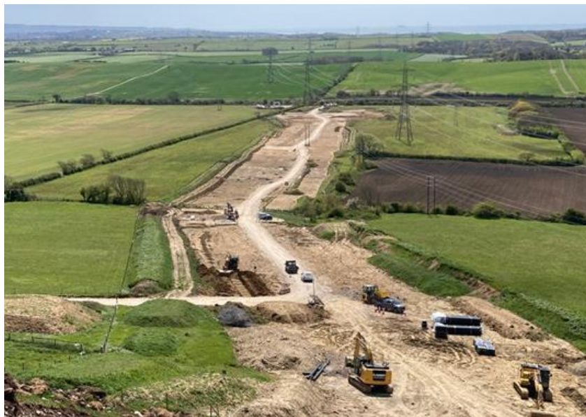
Figure 2.3 – Example Cable Construction
