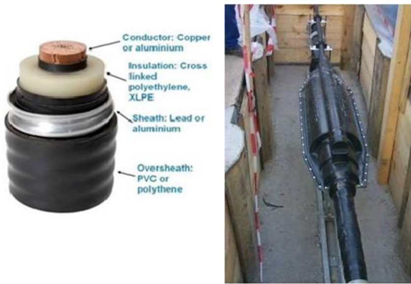
Figure C.4 – Cable Cross Section and Joint
