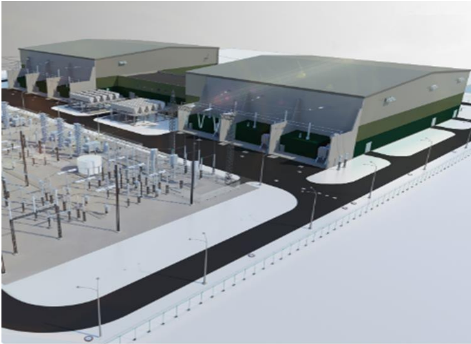
Figure C.7 – VSC convertor Station
