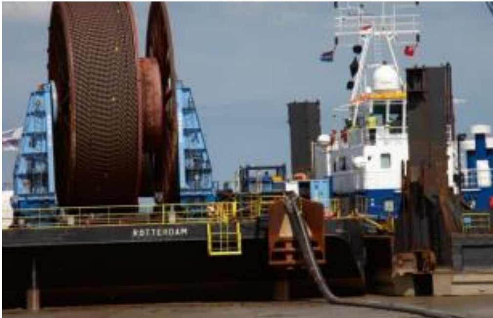
Figure C.8: HVDC Cable Laying Barge at transition between shore and sea cables
