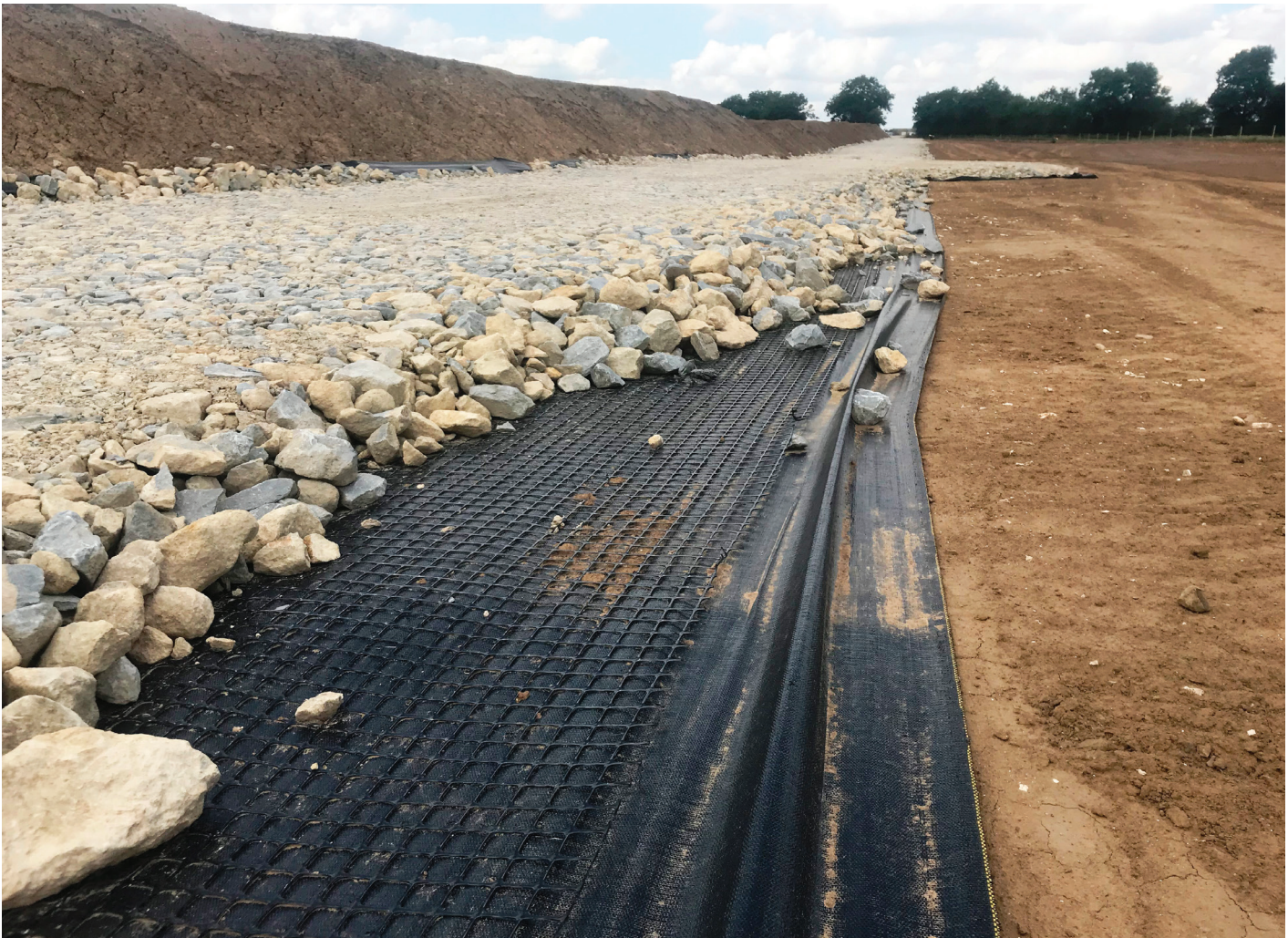
Construction haul road formation
