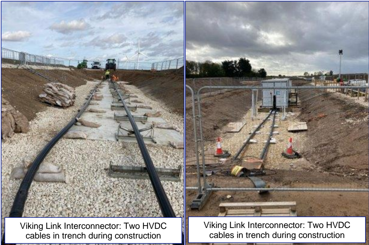
Figure 2-2– Example DC Cable Construction
