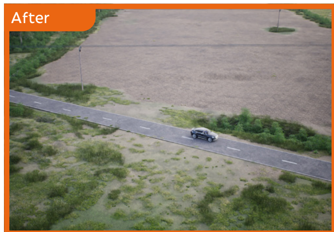
Images showing the cable route site prior to construction (TOP), during construction (MIDDLE) and six months post-construction (BOTTOM).
