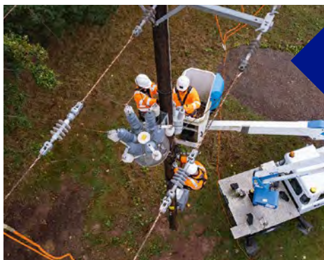
UK ED engineers undergoing training on maintaining pole mounted equipment.
