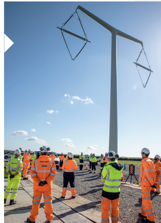
The first of 53 T-pylons, erected in September 2021 as part of the Hinkley Connection project in the UK
