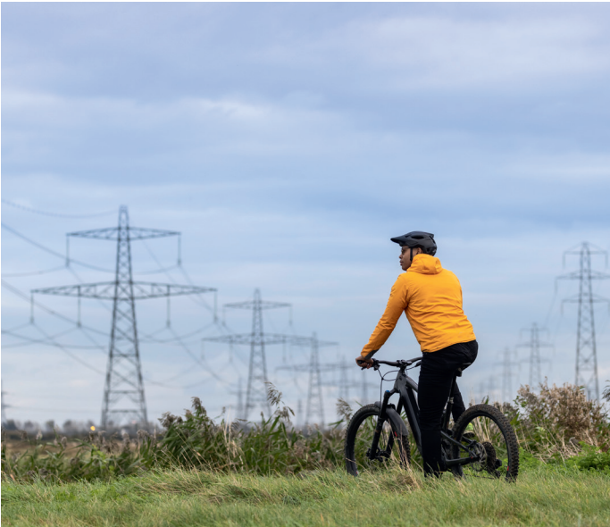
The Nemo Link Interconnector that runs between Britain and Belgium powers the Richborough and Canterbury, high-voltage overhead line.
