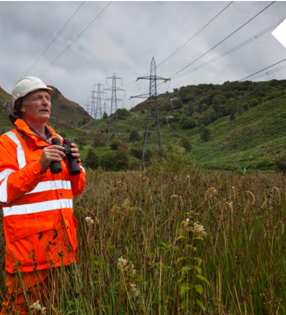
Overhead lines (OHL) inspection, from the ground, UK
