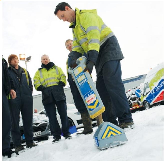
Cable avoidance in Gas Distribution
