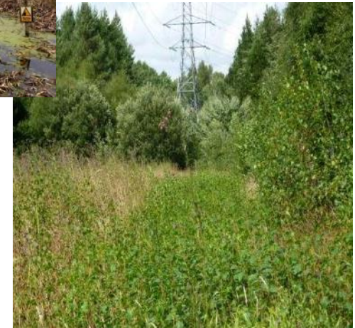
Overhead line 'V' profile
