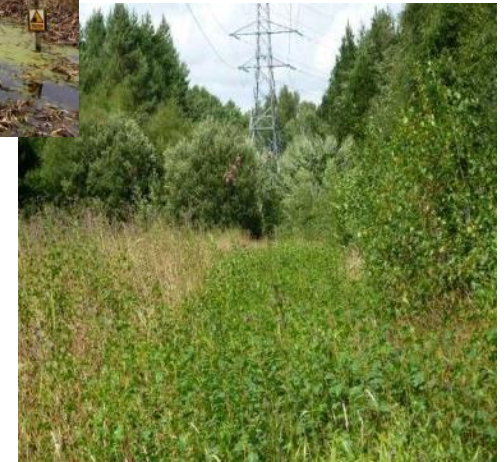
Overhead line 'V' profile
