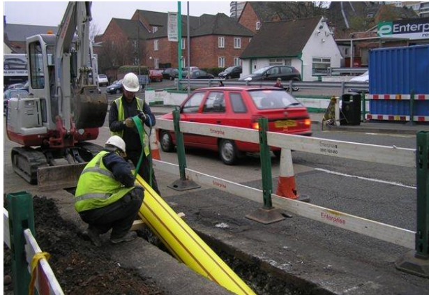
Gas mains replacement
