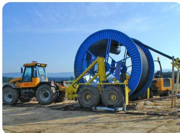
Left: Cable joint bay on a directly buried cable.
