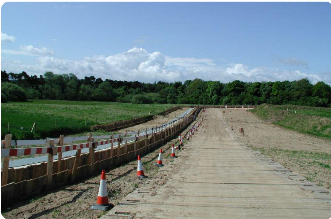
A cable swathe with a single cable trench open.
