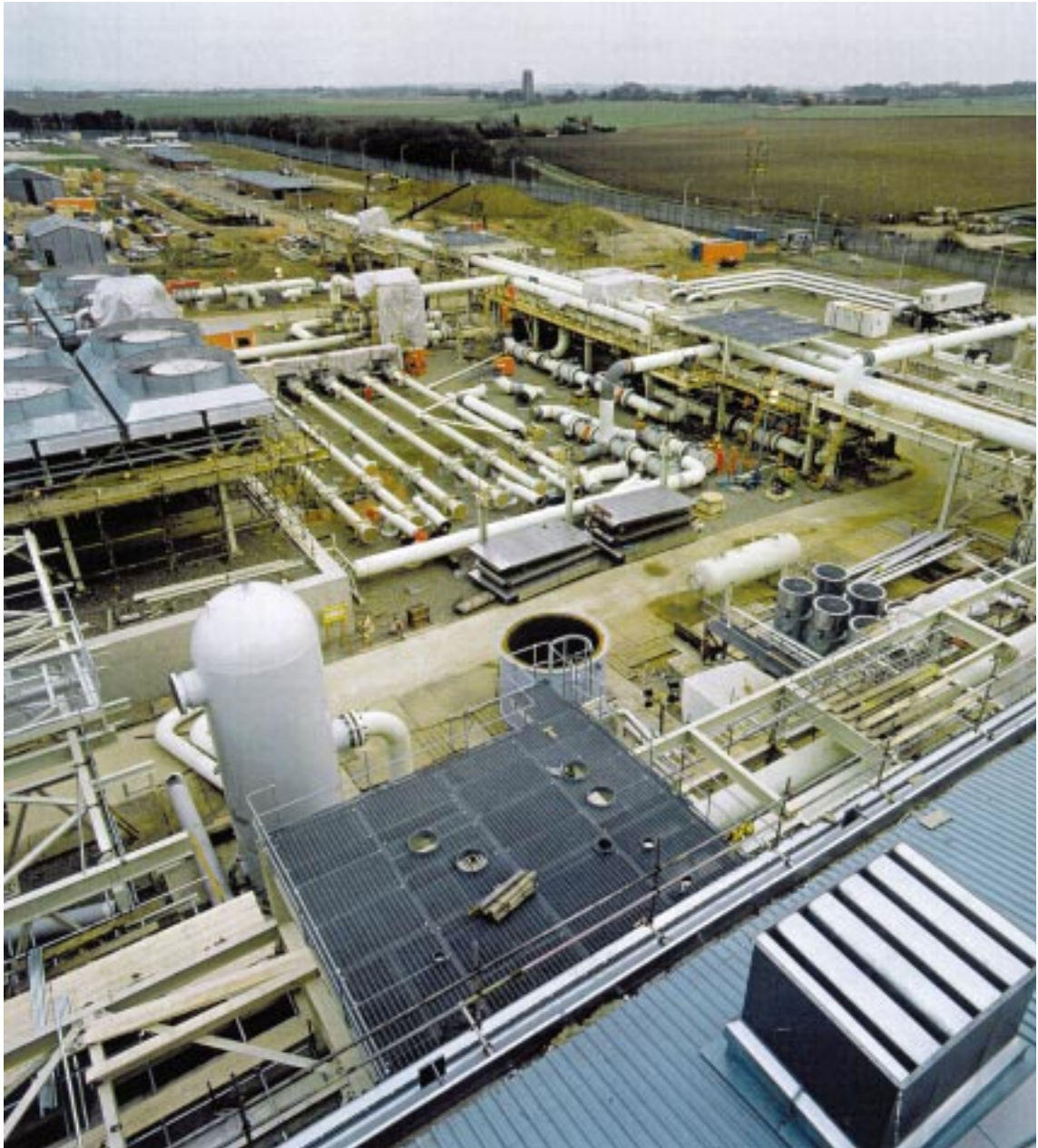
Figure A8.1.1b - Progress Photograph as at January 1998.
