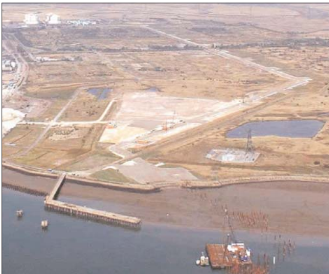
Figure 5 - Aerial view of Isle of Grain Construction
