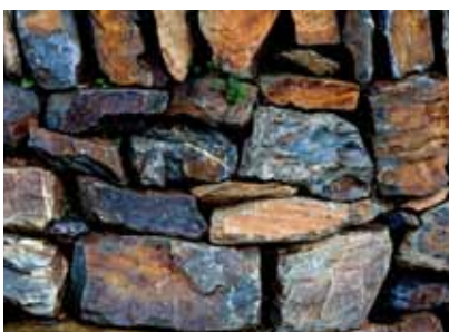
A reinstatement to a road crossing on the route of The South West Reinforcement Project. The breach was repaired using traditional Devon Banks methods.
