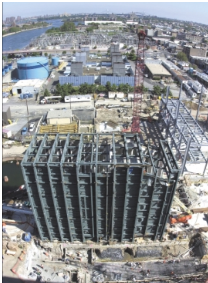
Construction is progressing on KeySpan's 250MW Ravenswood Expansion.
